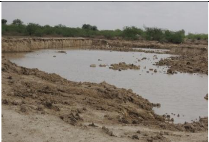
During the Pond digging by Connribution
