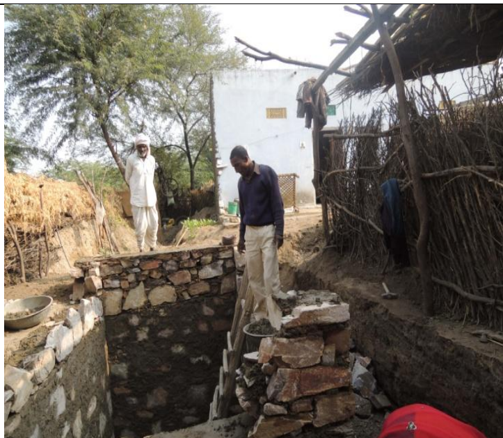
During Family Tanka Construction of Suva Ram Balai
