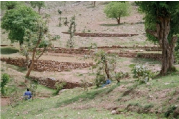
Gully plugs at Malawari
